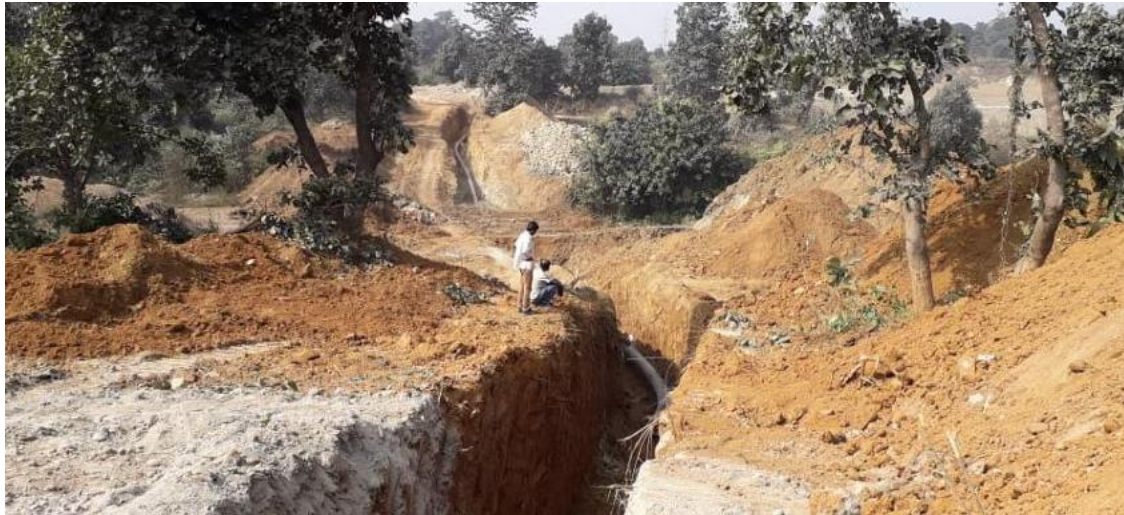
Pipeline laid for a Cross-Country Project
